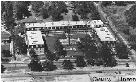
The Richelieu Apartments before Hurricane Camille
