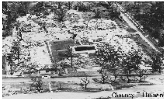
The Richelieu Apartments after Hurricane Camille
